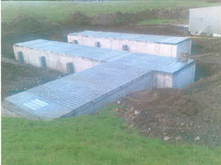
ict.mic.ul.ie Construction of a Slatted House
