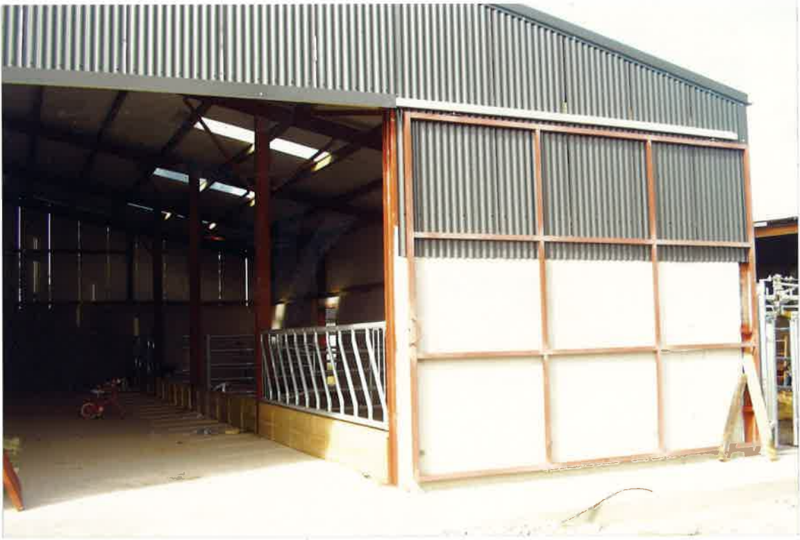
9. Here we see the frame of the sliding door as well as it's slide-ways.
